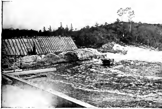
FIG. 11.—DAM, LEWISTON AND AUBURN, ME., PLANT.
